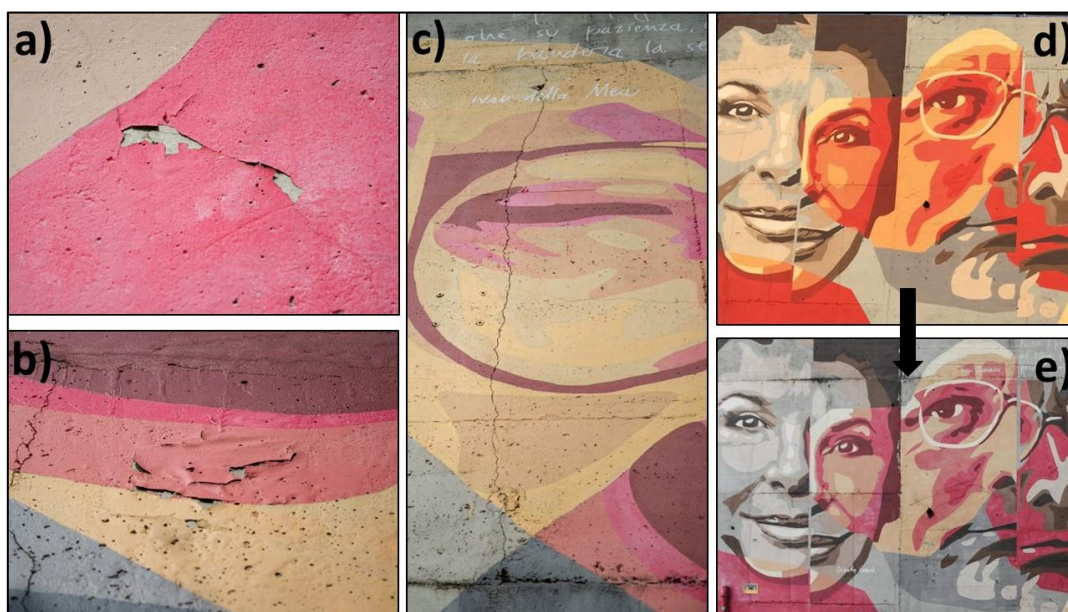
Figure 4. Images from the contemporary mural “Musica Popolare” by Orticanoodles (Milan, Italy): examples of deterioration patterns that can be observed on contemporary murals. (a) Flaking; (b) scaling; (c) fracture of the substrate; (d) original colour of the artwork realised in 2016 and (e) colour fading observed.
