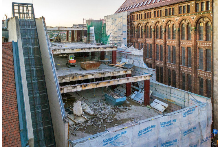
Figure 10. Demolition of the MVM-OVT, 2020 (Source: www.pestbuda.hu )
