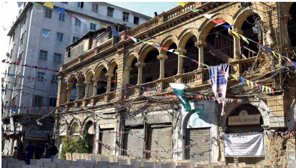
REGENERATION OF HISTORIC CORE, DENSO HALL RAHGUZAR WALKING STREET, KARACHI, PAKISTAN, 2019-2021 © HERITAGE FOUNDATION OF PAKISTAN
