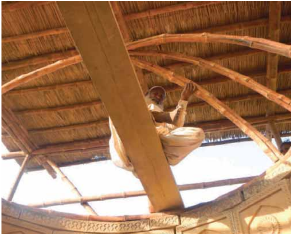
RESTORATION AND CONSERVATION PROJECT, SEPULCHRE OF MIRZA JAN BABA, MAKLI NECROPOLIS, PAKISTAN, 2014-2016 © HERITAGE FOUNDATION OF PAKISTAN
