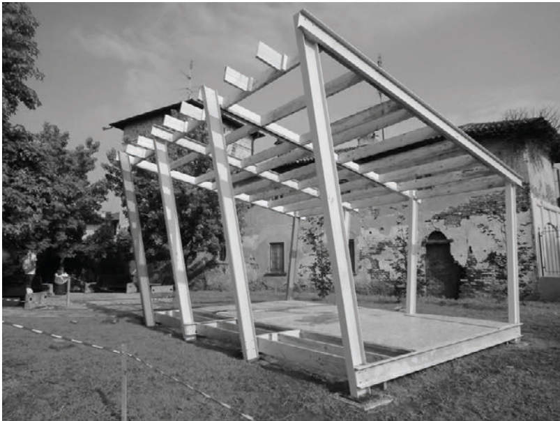
Figure 2. Module StONE, Abbiategrosso. Structural members in fibreglass coupled with timber elements using the Segal Method ([source: Alessandro Rogora]).
