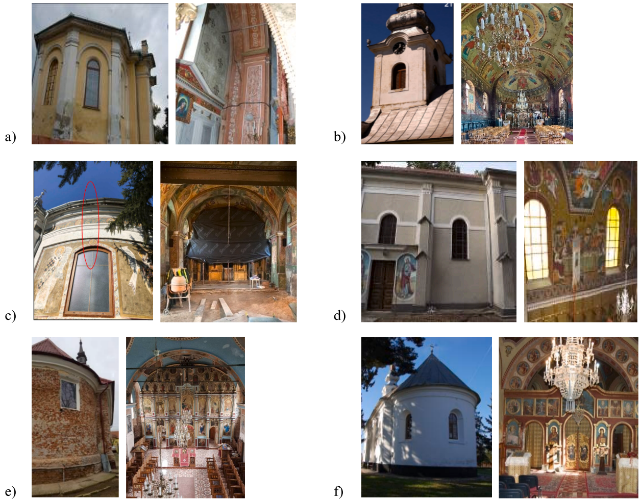
Fig. 4. Exterior and interior pictures which show the conservation state of the investigated churches: a) Holy Spirit Descent Church of Cenad; b) Virgin Mary's Nativity Church of Chizătău; c) Saint Nicholas Church of Bocea; d) Saint Nicholas Church of Bencecu de Jos; e) Saint George Church of Beregsău Mare; f) Jesus Resurrection Church of Belinț.
