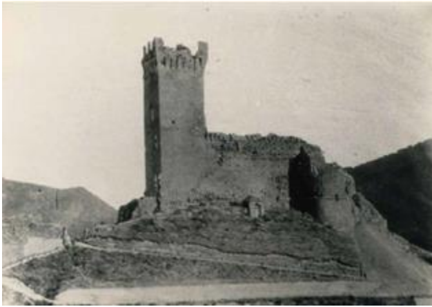
Fig. 7: Photo of the Stronghold (western facade) before the restoration works of the late 19 th century/beginning 20 th century (Istituto Centrale per il Catalogo e la Documentazione).
