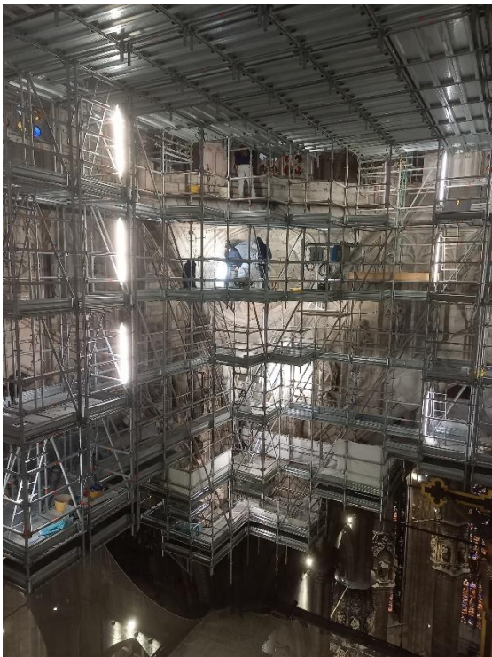
Figure 1 – The scaffolding for the Tiburio restoration
