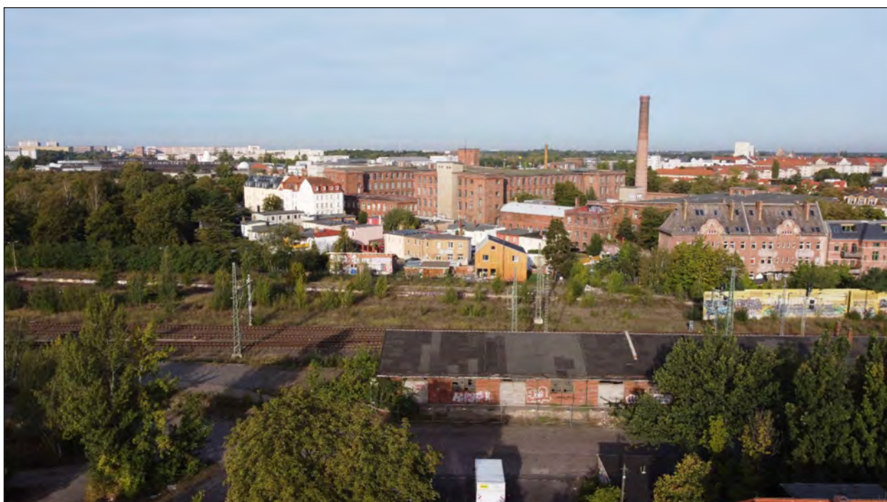
Figure 4. The restored Leipziger Baumwollspinnerei industrial complex next to the Bürgerbahnhof Plagwitz and Gestattungsvereinbarung, October 2021. Source: author
