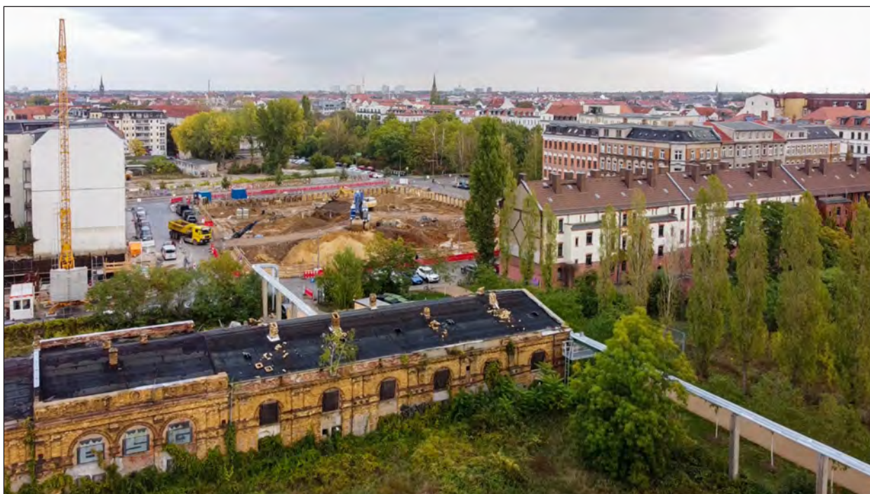
Figure 10. A construction site located near Lene-Voigt-Park and the Reudnitz-Thonberg district designated for the development of a residential complex. October 2021. Source: author .
