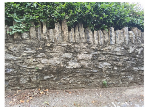
Fig.5 – Types of coping: 1 | Flat stones (above) 2. Standing stones (below). Case studies in Laglio (CO) (above) and Cenobbio, Rovenna (below). Illustration: Dani Pelagatti and Stiftung Umwelteinsatz, using in accordance with Creative Commons CC-BY-SA-4.0
