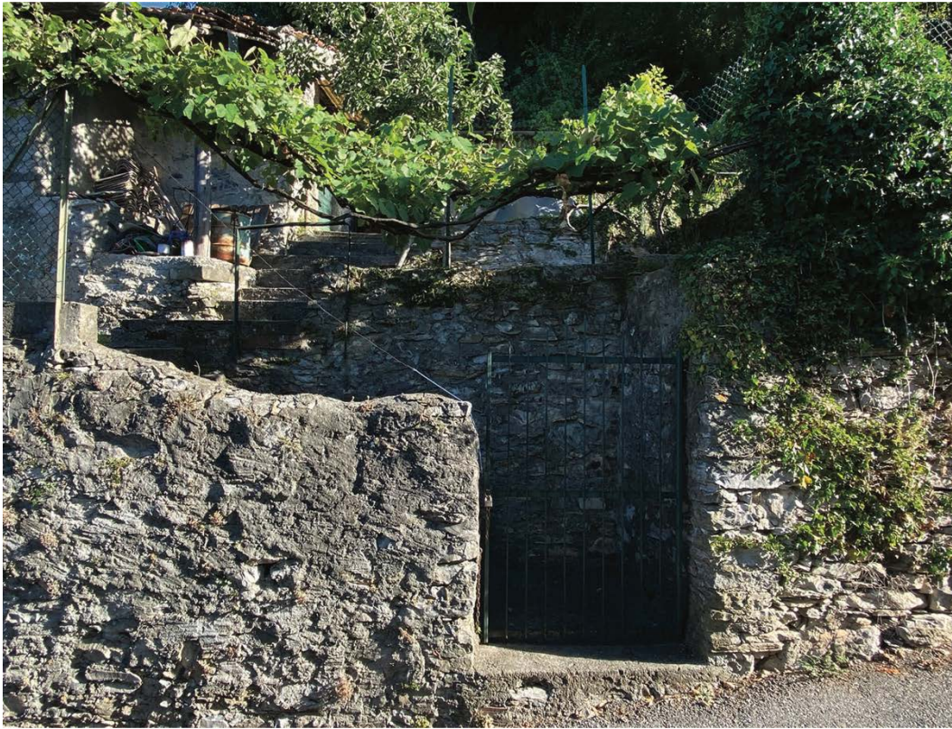
Fig.2 – A dry-stone walls included inside a familial urban garden. Cernobbio, Rovenna (Co)
