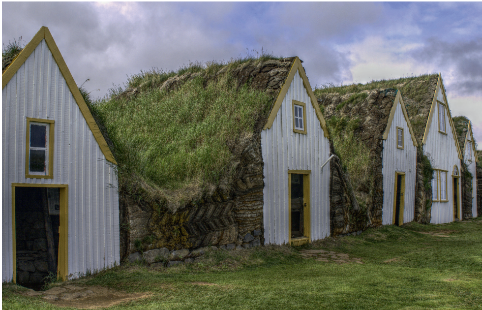
Figure 2. The characteristic turf houses of Iceland as a pioneer application of moss on buildings.
