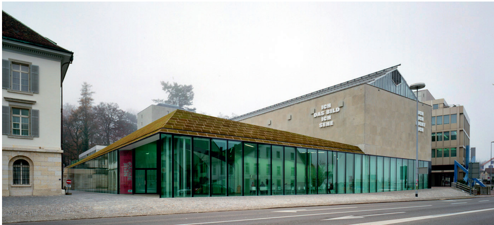
Figure 5. Expansion of the Fine Art Museum, Aarau, Switzerland (1998-2003), by Herzog & de Meuron, with moss cultivated directly on the tuff-like limestones of the roof.
