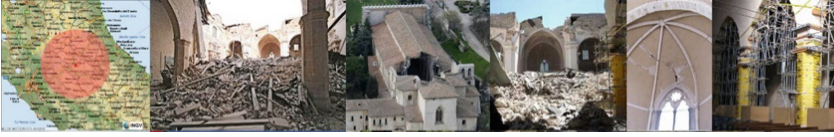
Fig. 1. The area struck by the earthquake at L'Aquila and the damaged Basilica di Collemaggio
