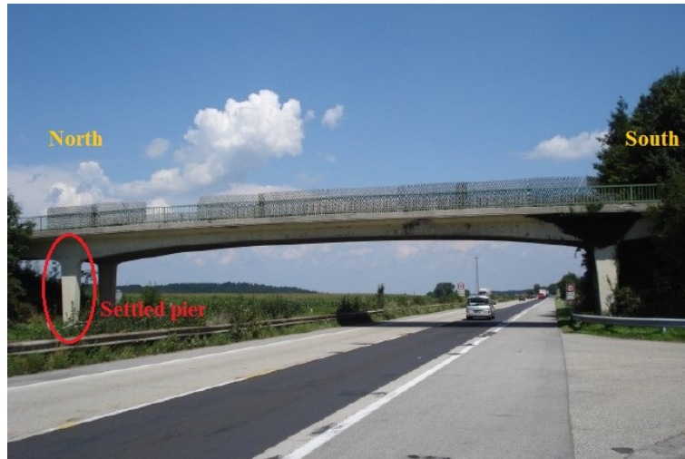
Figure 1: Lateral view of the bridge
