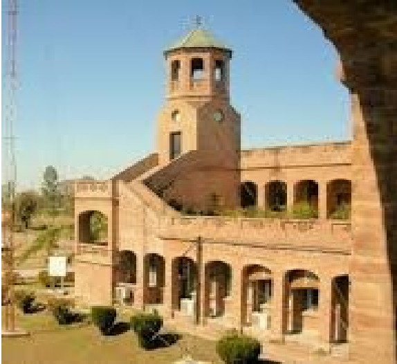
Fig. 8: Chand Bagh School, Muridke, 1997 (source: Chand Bagh School, https://chandbagh.com.pk/ )
