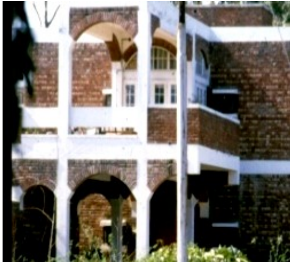
Fig. 4: Asad Qurban Ali Res, Lahore, 1980 (source: Kamil Khan Mumtaz Architects Archives)
