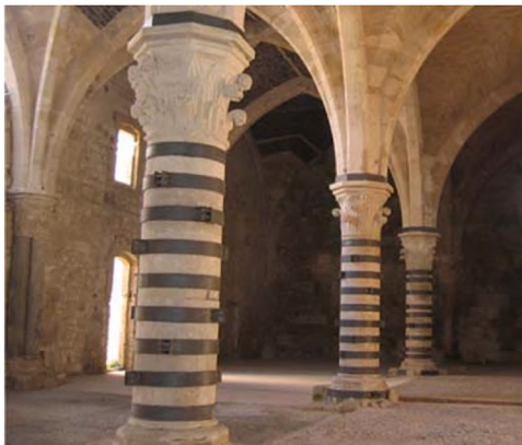
Fig. 3. Steel hoops on columns of the hypostyle hall in Maniace Castle in Syracuse, Italy.
