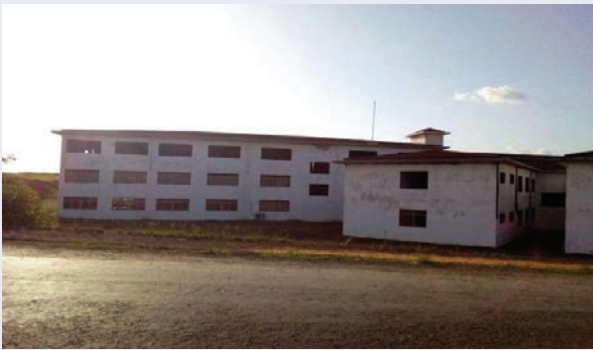
Bong Community College under construction
