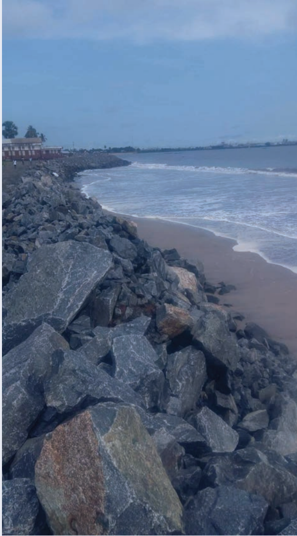
Building a coastal defence wall in New Kru town
