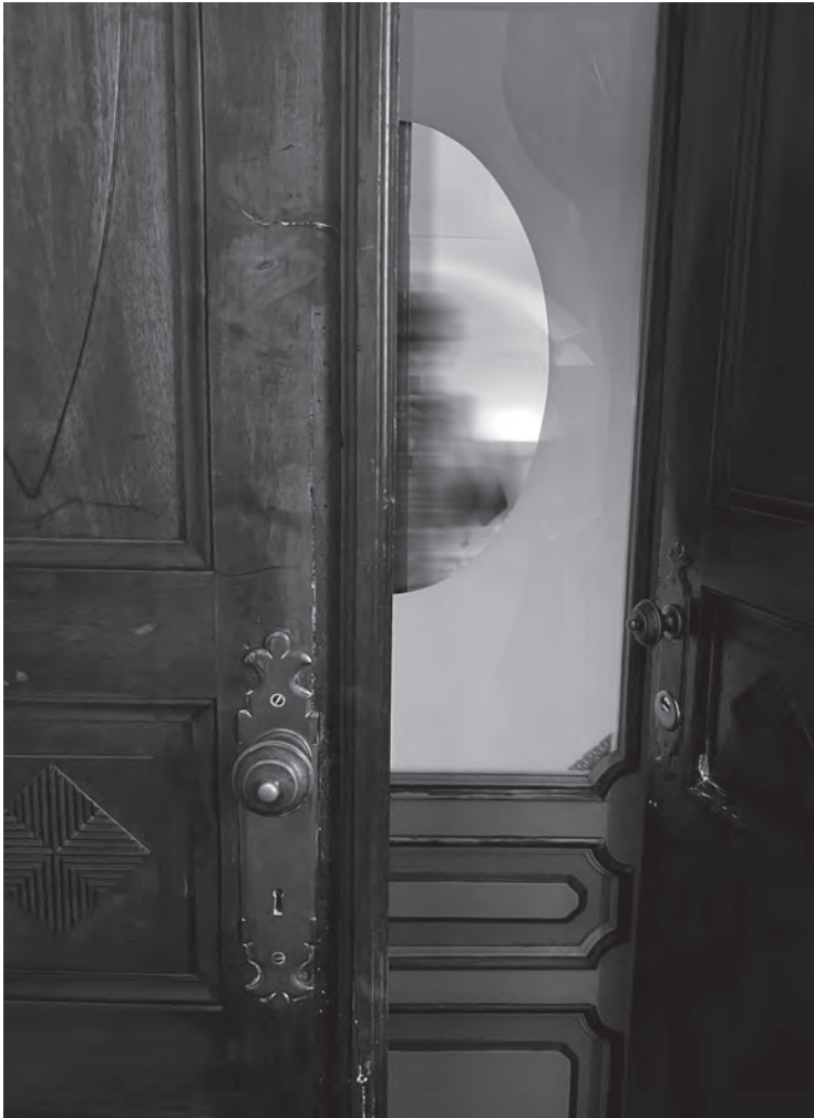
Casa Mollino, double-door entrance system. Photo by the author.
