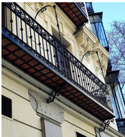
Figure 7. Fastening brackets and anchors to the wall of the continuous balconies
