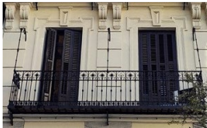
Figure 2. Continuous balcony. Calle Churruca 47.
