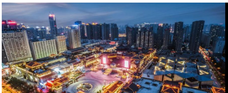
Figure 3. Aerial View—West Market of the Great Tang, Xi'an, opened 2012. (Adapted from gov.chinadaily.com.cn)
