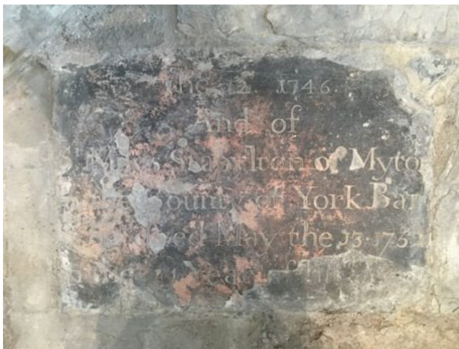
Figure 1. Example of ledger stone, with signs of delamination, by David Littlefield
