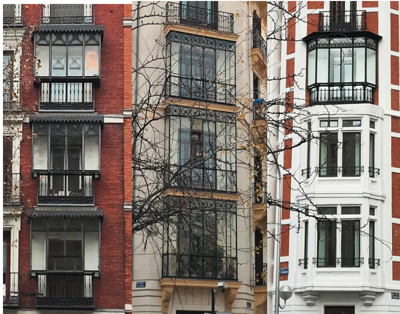
Figure 3. Bay window. Calle Carranza 24
