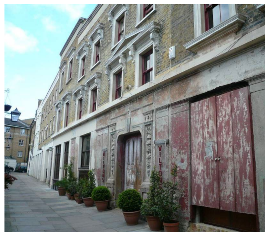
Figure 2. Graces Alley looking West
