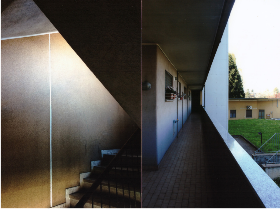
fig. 2. INA-Casa Neighborhood Harar-Dessiè, Milan, 1951-1955. Building Via Harar 3, G. Ponti, L. Ghò: staircase/distribution balcony. Photo sequence from the photoworkshop Everyday Architectural Heritage, © Architectural Preservation Studio – A. Canziani (2017), AUIC School, Politecnico di Milano
