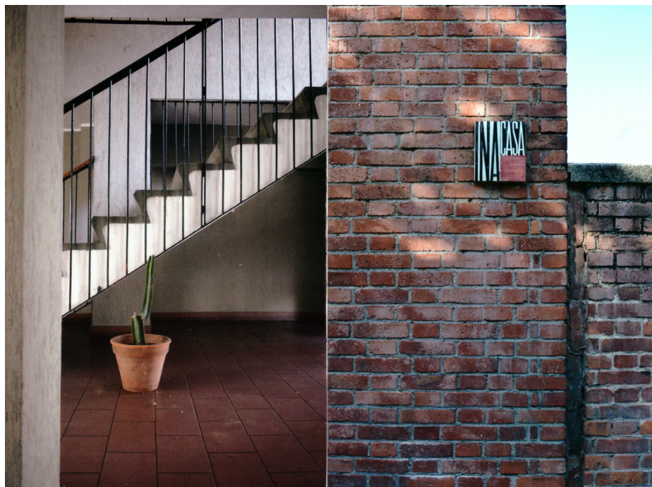
fig. 1. INA-Casa Neighborhood Harar-Dessiè, Milan, 1951- 1955. Building via Dessiè 15, M. Tevarotto, G. Reggio: staircase / Insulae Via Varenna, L. Figini, G. Pollini: external wall. Photo sequence from the photoworkshop Everyday Architectural Heritage, © Architectural Preservation Studio – A. Canziani (2017), AUIC School, Politecnico di Milano
