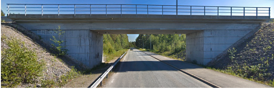
Fig. 10. Hörnefors railway bridge.
