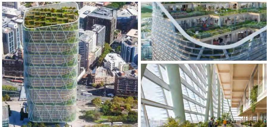
Figure 22. Mass Timber Construction (MTC) at Atlassian HQ Sydney towards net-zero carbon emissions (D’Angelo, 2020).
