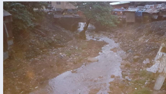
Kissy Brook Bridge after the FCC clean up
