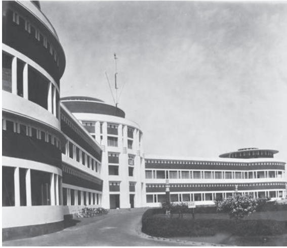
Figure 5a.3 Photograph of All India Old Broadcasting House in New Delhi, c. 1930 Source: The Central Public Works Department.
