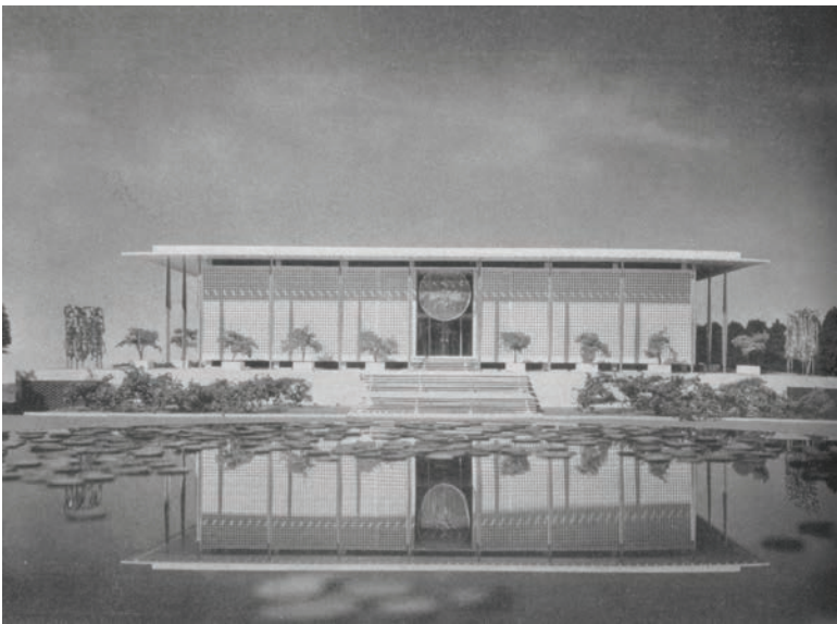
Figure 5b.20 Photograph of the US Embassy, c. 1953
