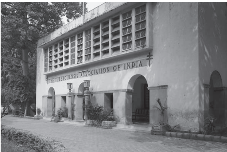
Figure 5b.28 Photograph of the Tuberculosis Association of India Building in Delhi, 2014 Source: Author.
