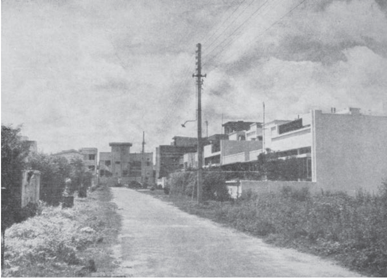
Figure 4.15 Photograph of Defence Colony after Independence, c. 1960 Source: The Indian Architect (1962: 22).
