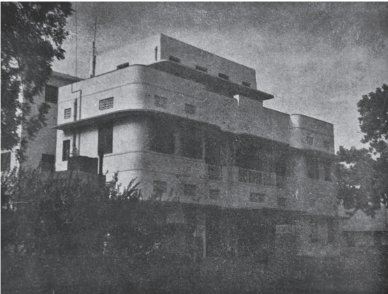
Figure 3.7 Photograph of One of the Houses in Daryaganj, c. 1925 Source: Central Public Works Department, Delhi.
