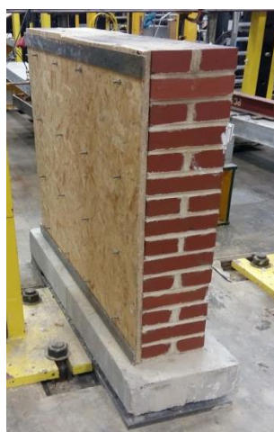
1-sided retrofitted wall
