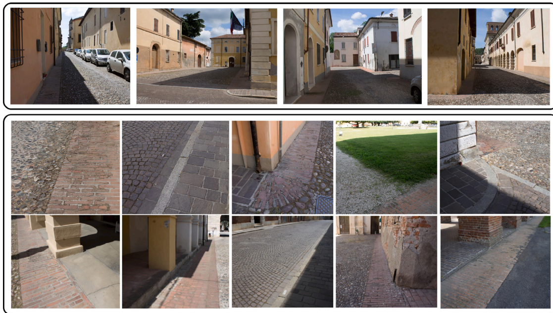
Fig. 12. Photos of the city of Sabbioneta, a case study for this paper. (a) Views of some streets in the city. (b) Layering of different pavements used for different elements of the urban area in the city, sidewalks and roads are highlighted by the use of different paving materials.
