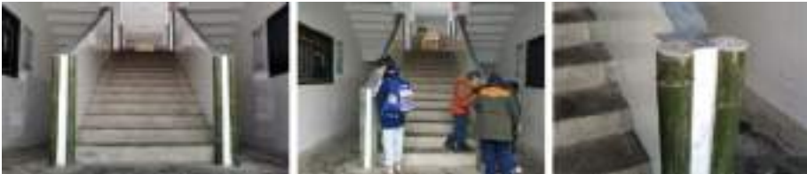
Fig. 6. Anti-collision bamboo pile
