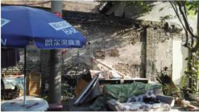
Fig. 3. The alleviated and renovated Paoju Toutiao Hutong with residents' items, Dongcheng District. (By Huan Wang)
