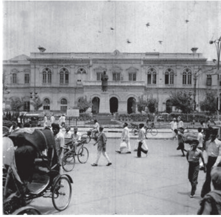
Figure 5a.13 Photograph of the City Hall in Old Delhi, 1930 Source: Delhi State Archive.
