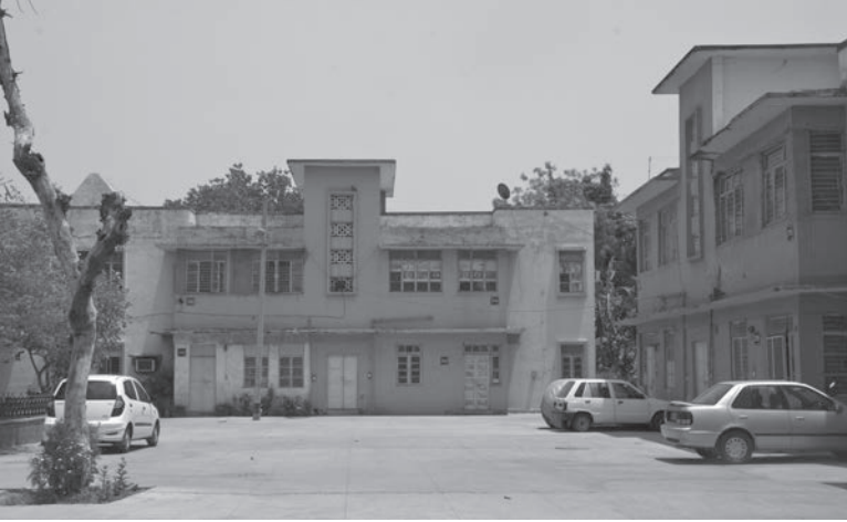
Figure 3.15 Photograph of One of the Modern Houses of Laxmi Bai Nagar Colony Built Immediately after Independence, 2014
