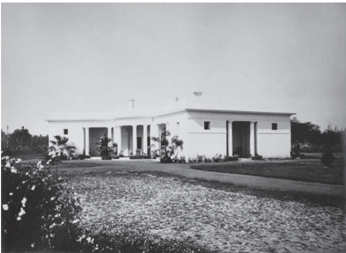
Figure A.18 Photograph of One of the Many Bungalows with 'Classical' Features in New Delhi, c. 1928 Source: Central Public Works Department.
