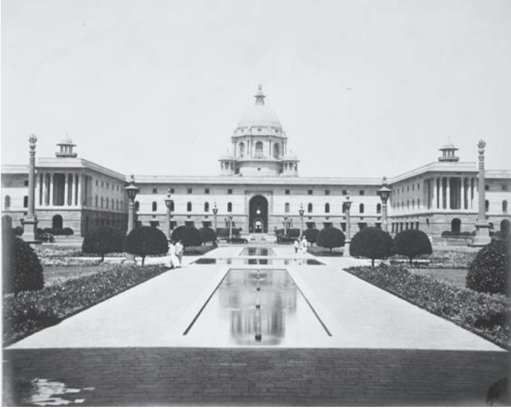
Figure 5a.7 Photograph of the Rashtrapati Bhavan in New Delhi, c. 1931 Source: The Central Public Works Department.
