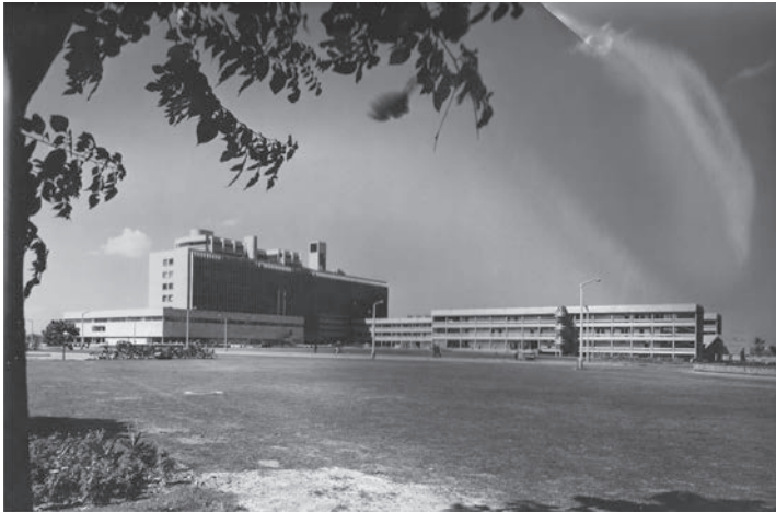
Figure 5b.4 Photograph of the Indian Institute of Technology, c. 1959 Source: Design (1969: 13).
