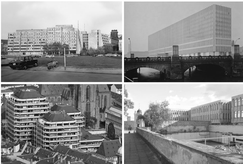
Fig. 3 Demolitions (from top left): Police Headquarters, Dresden; Foreign Ministry, Berlin; Technical Town Hall, Frankfurt a. M.; Teacher Training Institute, Potsdam.
