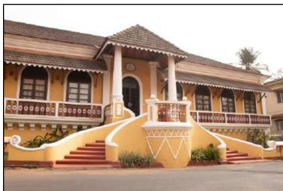
Figure 25. Balcão with Western-style columns connected to a semi-open passageway (Source: Lester Silveira, 2020).
