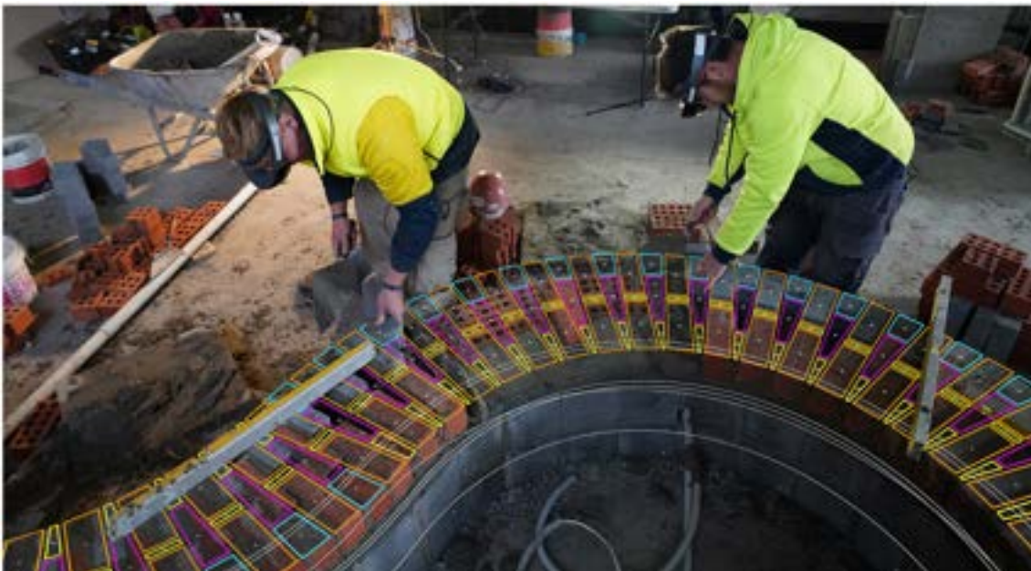
Figure 2 Mixed Reality App and Plugin for Design and Construction, Fologram
