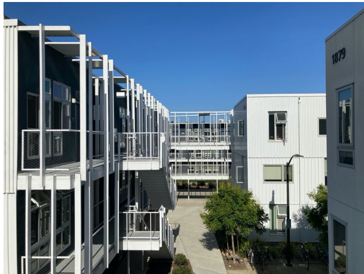
Figure 5. San Joaquin Student Housing Complex at the University of California Santa Barbara has all open-air circulation, with unit windows facing communal courtyard spaces.
