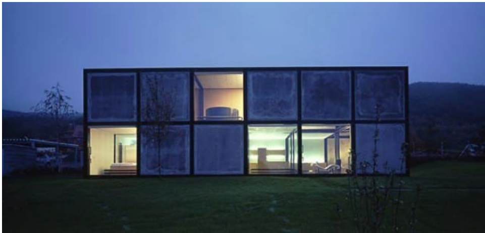
Figure 1. Villa in Beroun's outside view.
