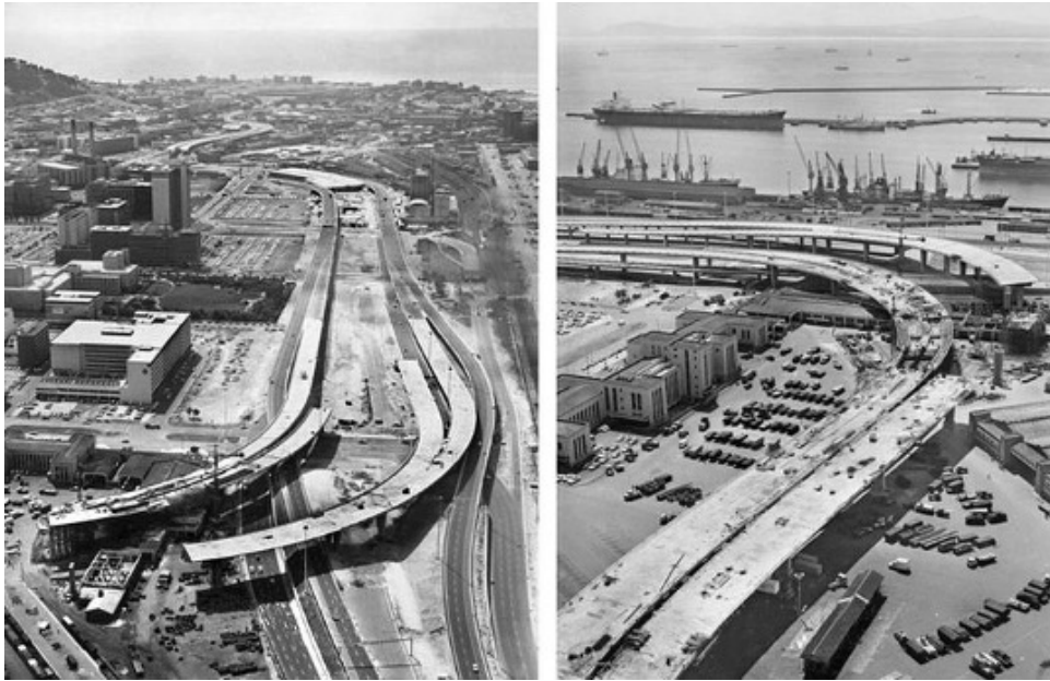
Figure 5. Foreshore highway under construction, 1970's. Source: http://digitalcollections.lib.uct.ac.za/collection/islandora-15123
