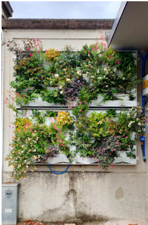
Figg. 2 and 4 (left side) and 3 and 5 (right-side). Respectively, Building 9 and 10 (B9-B10) and different configuration. The modules can be hanging with no limits in height, allowing the designer to adopt it to the building envelope.
