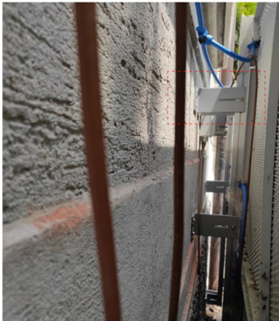
Fig. 10 (left side) shows (red hatched focus) the position of the AirCare sensor and the main components of the irrigation system.
