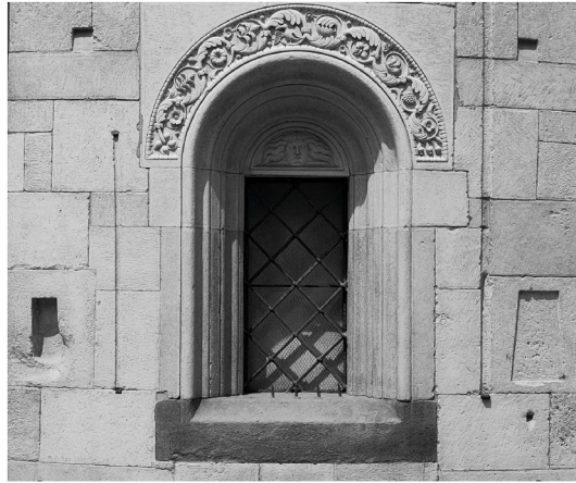
Figure 7 Recesses on the apse of Modena Cathedral (Italy); to the left of the window, those used to standardize/measure the dimensions of bricks; to the right, those used to standardize/measure the dimensions of roof tiles (authors' photograph)
