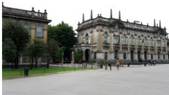
Fig. 1 Politecnico di Milano Building 3, where the AC PMD is hosted.
