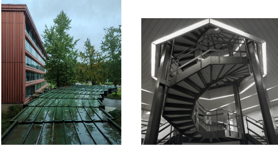
Fig. 4, 5. On the left: the view of the frontal canopy from above (source: K. Tafaro and R. Farahbod, 2025). On the right: the central octagonal staircase (source: Rossi Prodi F., 1996).
