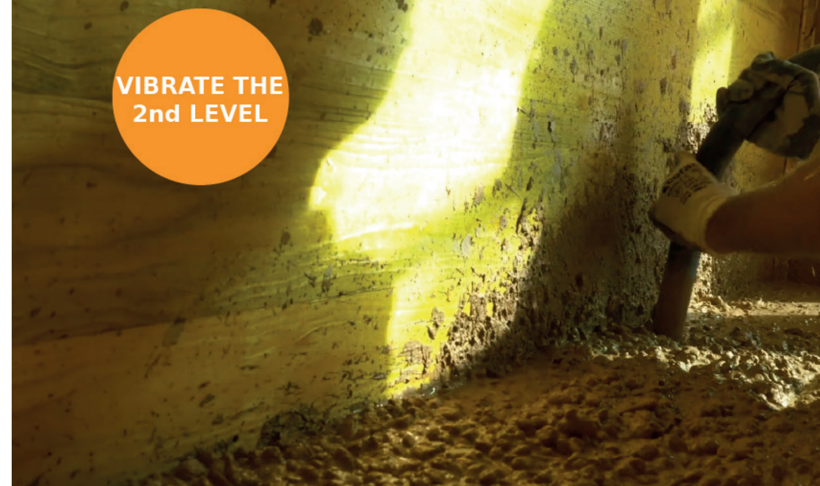
Video Tutorial by Bi0n. " Formwork Assembling - Poured Earth 2"
