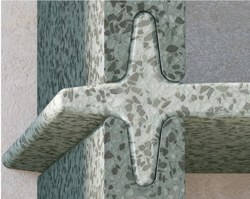
Detail of the star joint.
