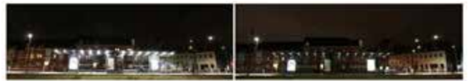
Figure 2. Photos a showing the existing bright lighting setting (left picture) and the dimmed lighting setting (right picture) at the Nørreport tram station, Aarhus.
