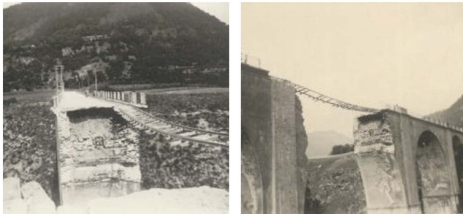
Figure 2. The collapse of the central arch occurred in 1944.
