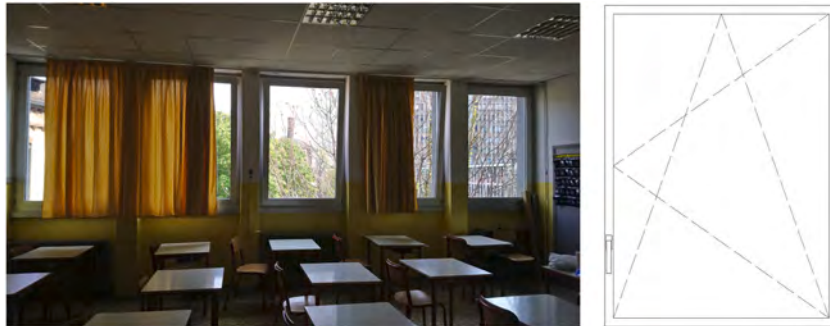
Fig. 6. Shape and typology of the windows found in classroom C3D. Type C: Tilt-and-turn windows with one casement.
