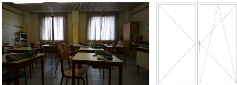
Fig. 4. Shape and typology of the windows found in classroom A1C. Type A: tilt-and-turn windows with two casements.
