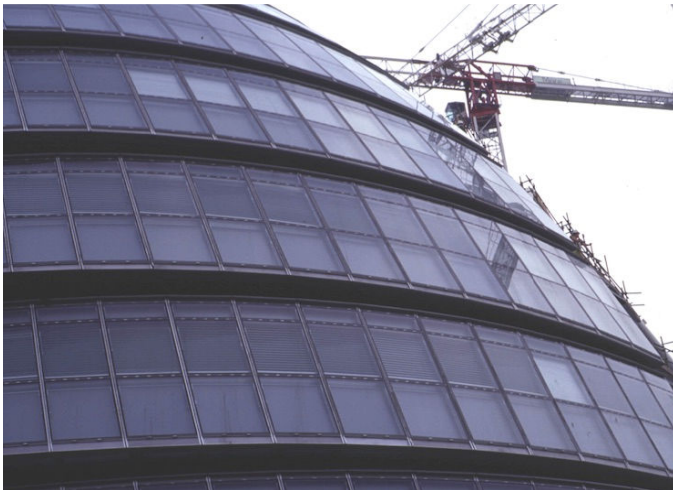
Fig. 16. Norman Foster and Partners, Greater London City Hall , London (©by the Author).
