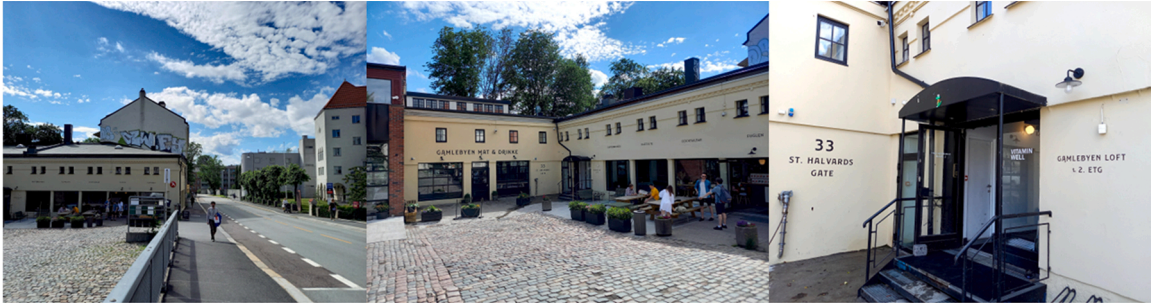
Fig. 13. The exterior of Gamlebyen Loft. Authors' pictures.
