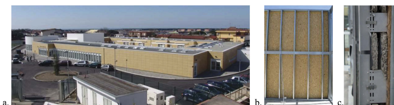
Figure 1. British Force School (BFS): a. general view; b. typical wall; c. external wall stratification.
