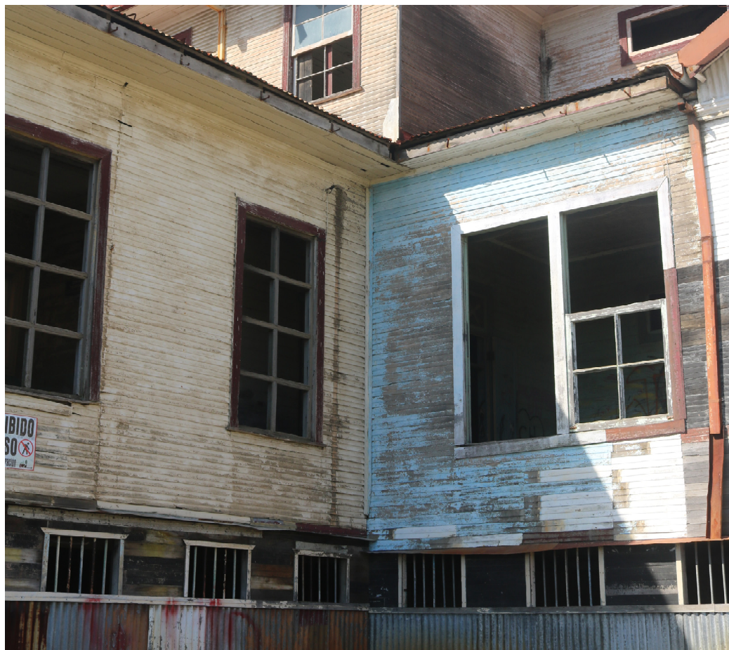
Figure 1. Physical Value of the Administration Building.
