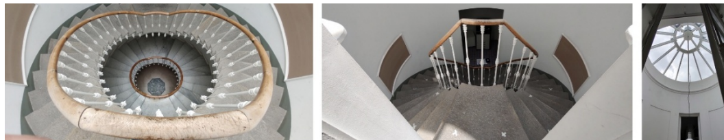
Fig. 5 – Photographic documentation of the main stairwell
