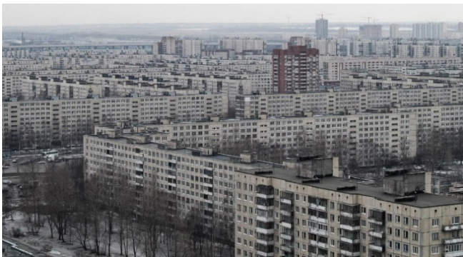
Figure 3. Kupchino District, Saint Petersburg (1970s housing development), Russia 1
