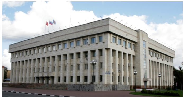
Figure 10. “White House” (City Administration Building), Lyubertsy, Russia 2
