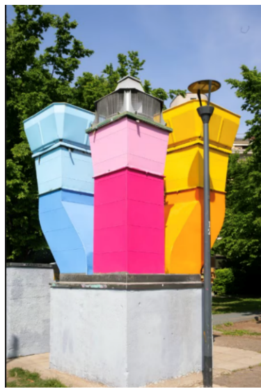
Fig.5_ Left_ cube shape structure for exit of underground parking. Previously abandoned and totally covered with unplanned doodles.
