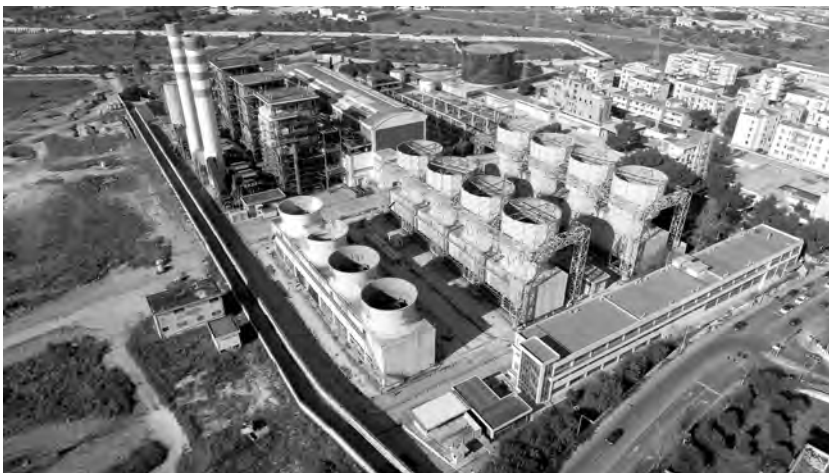
FIGURE 14.6 The power station of Bari, located close to the dismantled Stanic Refinery. Source: Enel Produzione S.p.A.
