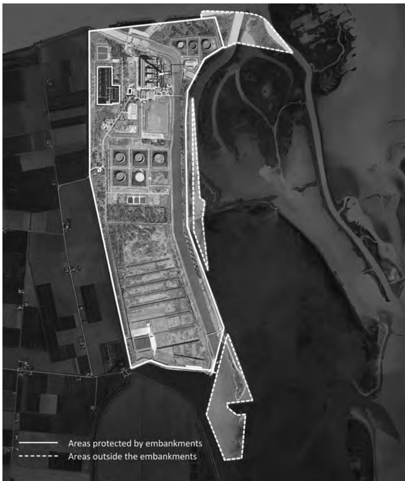
FIGURE 14.7 The power station of Porto Tolle. Source: Google Earth. Image © 2016 TerraMetrics – Data SIO, NOAA, US Navy, NGA, GEBCO modified by the authors.
