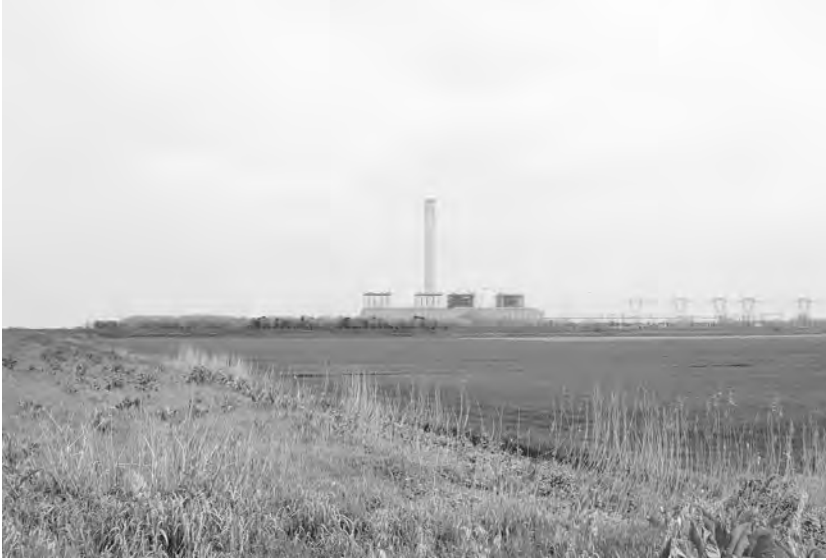
FIGURE 14.13 Porto Tolle power station. Source: Chiara Geroldi.
