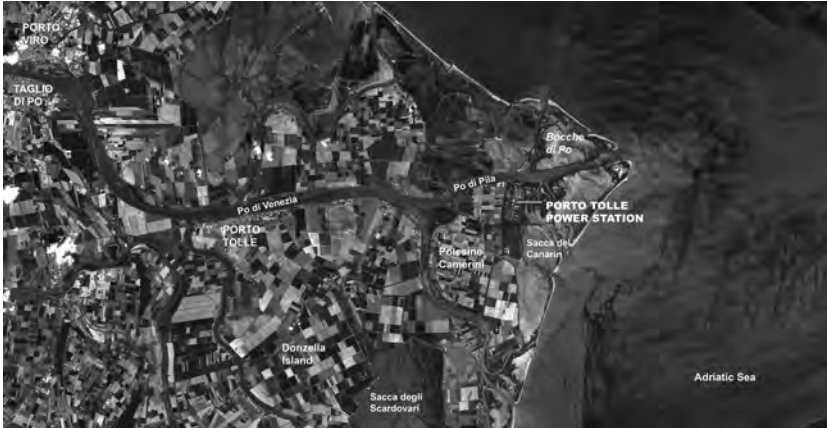
FIGURE 14.8 The power station of Porto Tolle in the context of Polesine (Po River delta). Source: Contains modified Copernicus Sentinel data (2020) (texts added by the authors).
