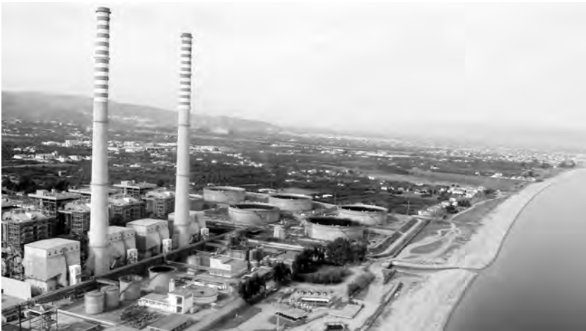
FIGURE 14.5 The power station of Rossano, located on the Ionian Sea. Source: Enel Produzione S.p.A.
