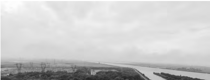
FIGURE 14.14 Electric station and system of pylons extending from the power station. Source: Chiara Geroldi and Gloria Pessina.
