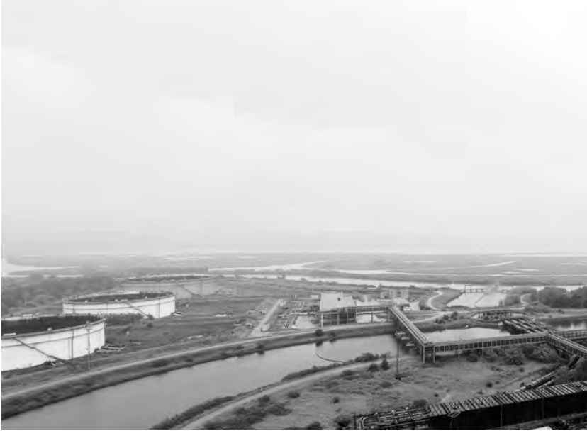
FIGURE 14.15 Oil tanks and view of the two canals used for plant cooling. Source: Chiara Geroldi.
