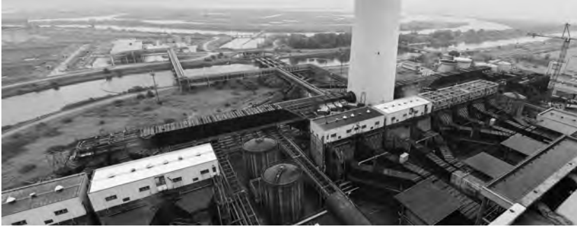
FIGURE 14.17 Intricate system of tubes and pipes in the proximity of the chimney. Source: Chiara Geroldi and Gloria Pessina.
