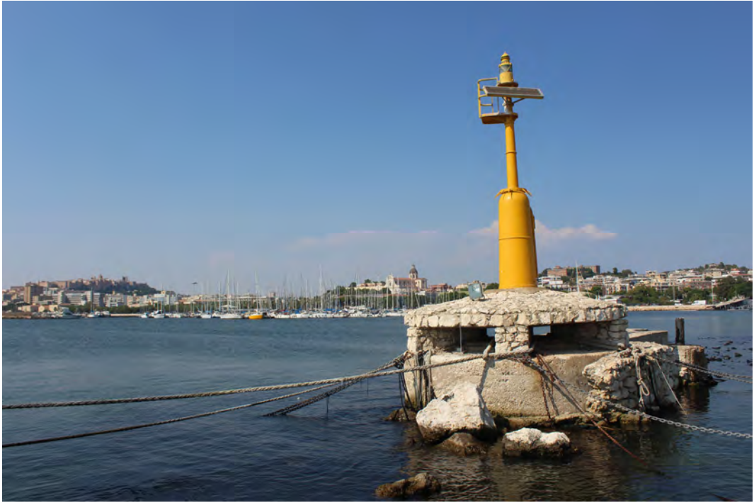
Fig. 5 Bunker number 93 in the Sant'Elmo pier. Giulia Cherchi
