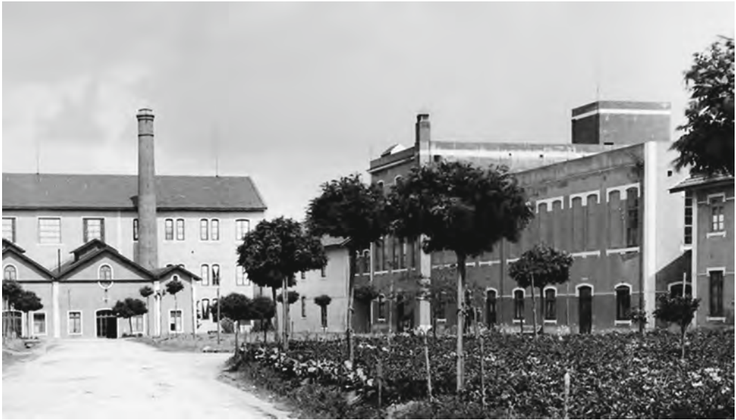
Fig. 4 Enlarged detail of the photograph. In the background, with the chimney, the original flour mill building; on the right the pasta factory. Exterior of the Leões Factory,
