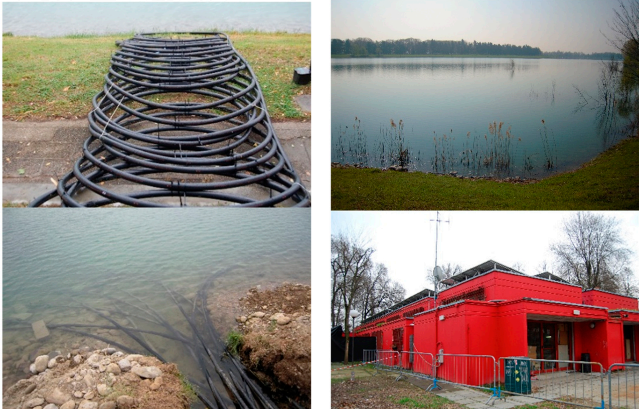
Figure 2. Thermal exchange system using the Idroscalo lake as a renewable heat source.
