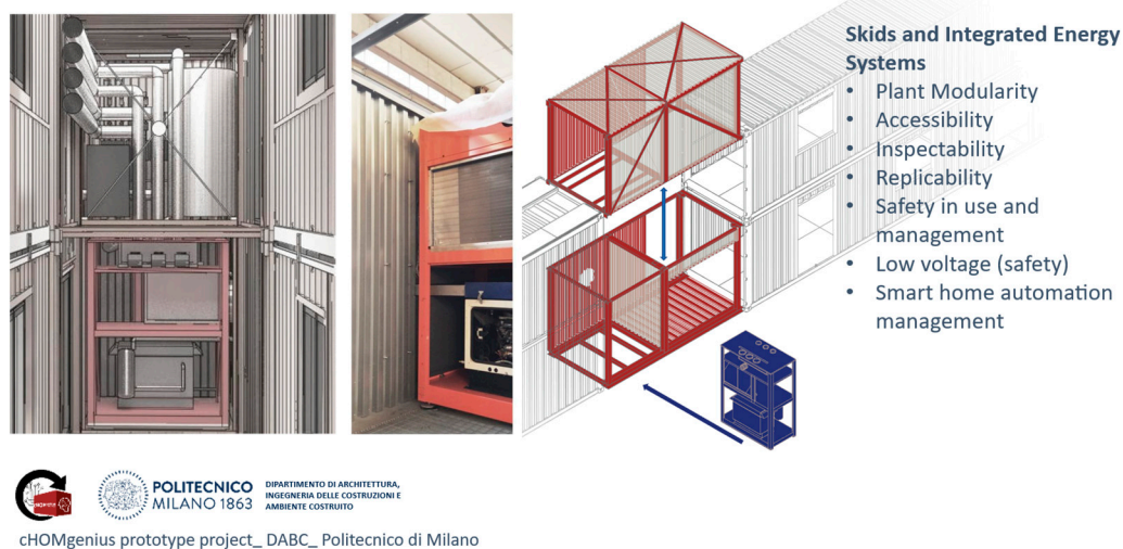
Figure 5. Integrated energy skid and modular plant system of the cHOMgenius prototype.
