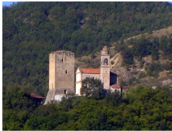
Figure 1. View of the tower.
