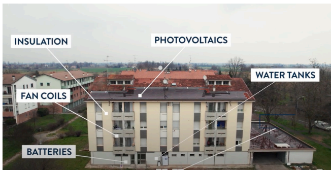
Fig. 3. View of the building after the retrofit process.
