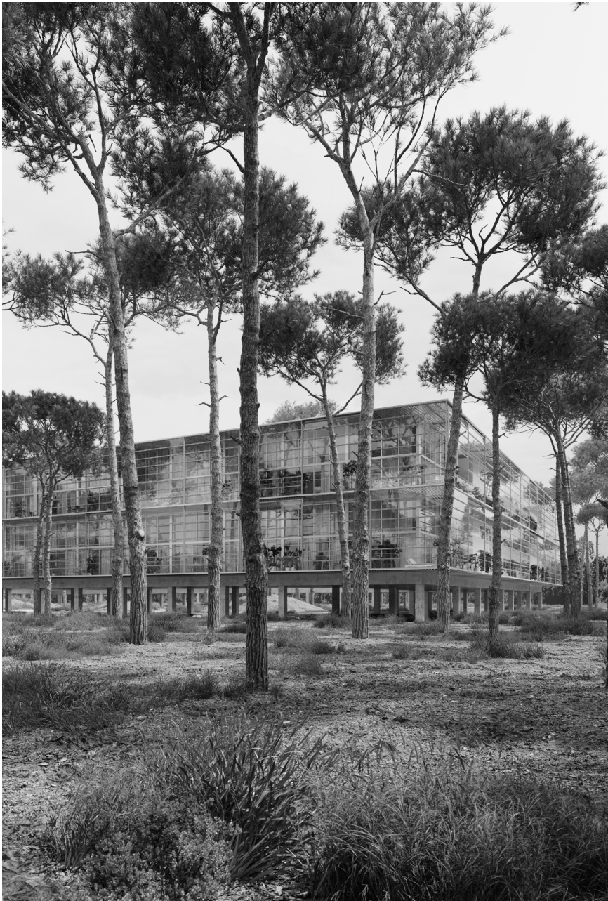
Bruther architectes (Stéphanie Bru, Alexandre Theriot), 160 Housing Units and One Parking, (Super-L), Eysines, France, 2013. BRUTHER © Photo by ArtaFactory Lab.
